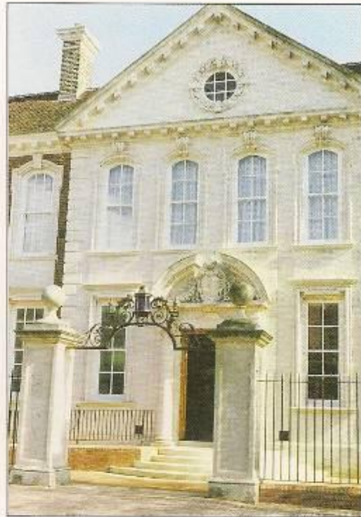
Front entrance to the police station
