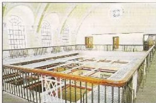
View of the newly renovated first floor balcony
