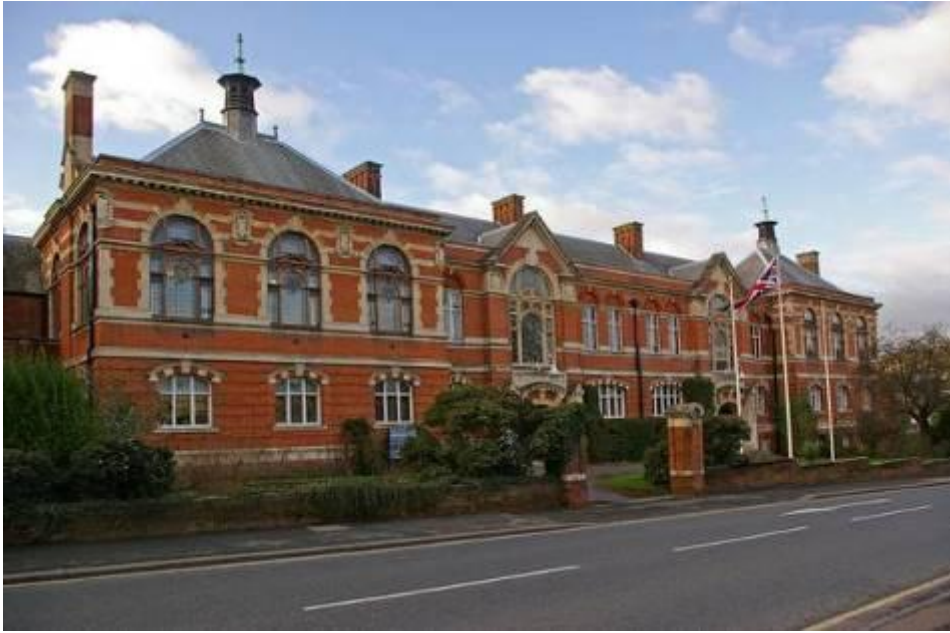
Reigate Municipal Buildings, housing the Town Hall on the left with the police station and court on the right side
