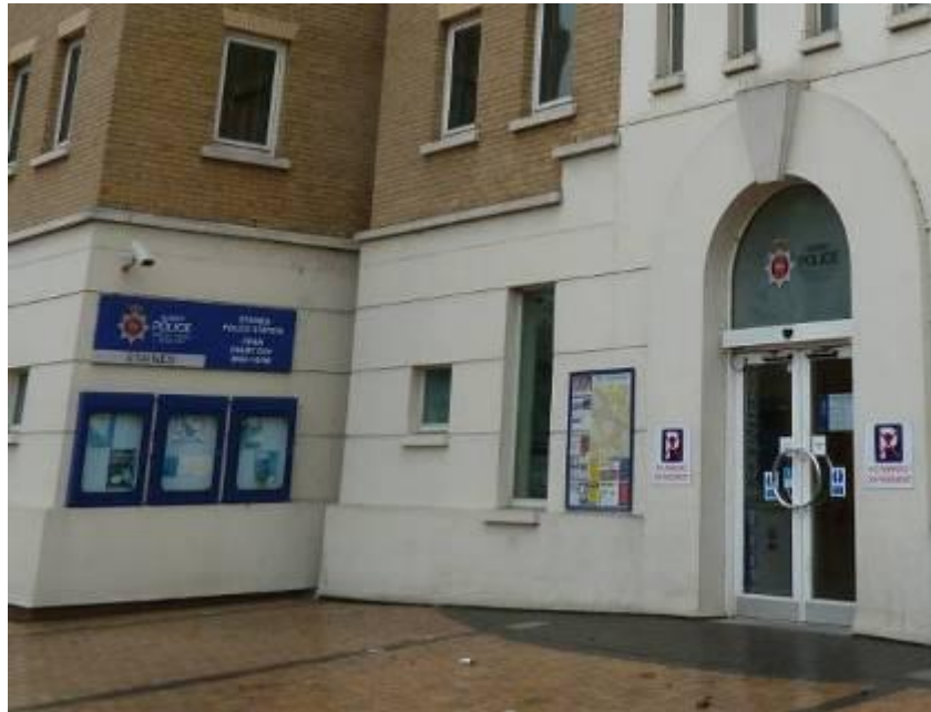
Staines: Haden James February 2011
