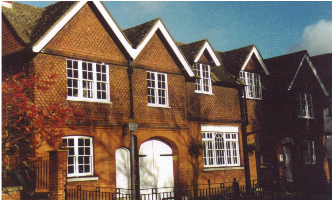
The room above the central arch of what was once the police station that became the magistrate's court is easily identified
