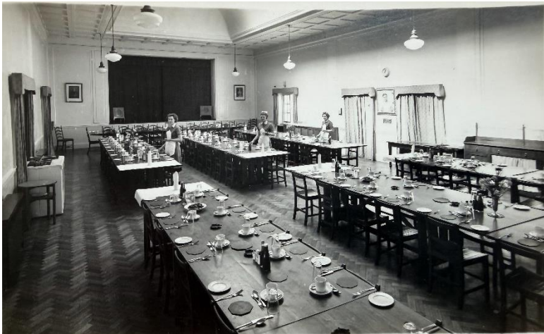
No. 6 Centre Dining Hall and stage which was severely damaged by fire in 1968
