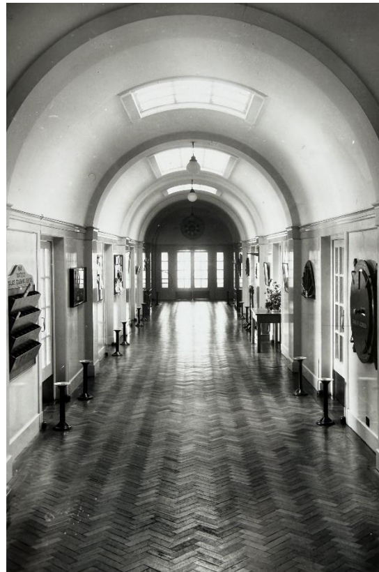
Sandgate Centre corridor to class rooms
