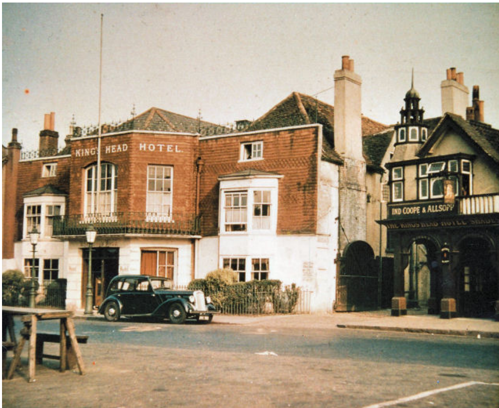
Epsom's first major building, the Kings Head dominated the High Street until it was pulled down for shopping in 1957.
