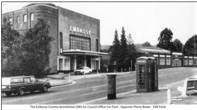
The Embassy Cinema demolished 1983 for Council Office Car Park - Opposite Phone Boxes - K49 Point
