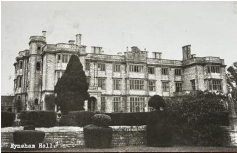
Eynsham Hall No. 5 Police District Training school near Witney Oxfordshire.
